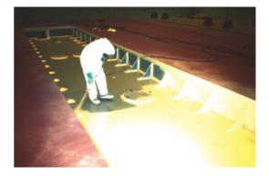
The PowerSpray works with servo-hydraulically actuated piston pumps with integrated distance measuring. The pump stroke is permanently superintendend and processed quantity and the mixing ratio will be varible controlled. Programmable "jumps" of the metering pumps at the commutation points reacting against the typical pressure release of the piston pumps and afford an optimal view of spraying by shortly pot-life time and extremely mixing ratios.
